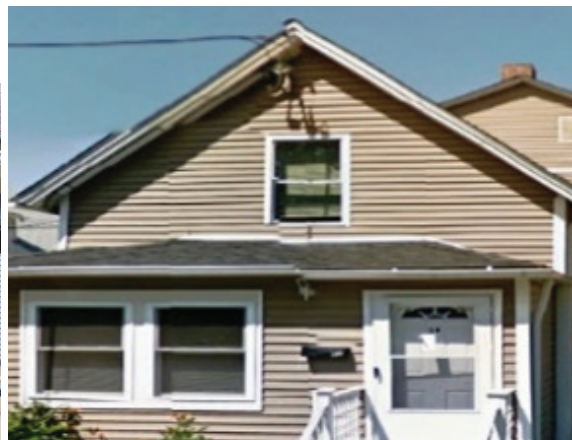
BEACON I STAMFORD OPENED: 2007 INDIVIDUAL UNITS: 5
