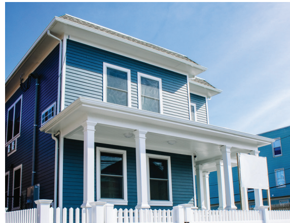
PARKVIEW NORTH (FRONT) NORWALK OPENED: 2021 INDIVIDUAL UNITS: 12
