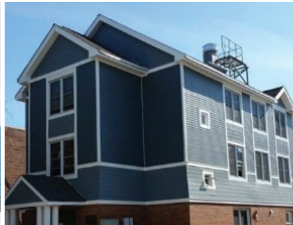
PARKVIEW SOUTH (REAR) NORWALK OPENED: 2015 INDIVIDUAL UNITS: 24
